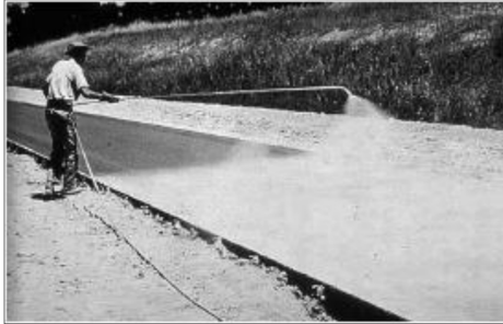
Application of liquid-forming compound with hand sprayer.
