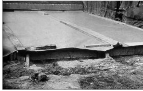
Slab-on-grade covered with waterproof paper for curing
