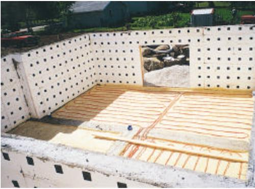
As a greater number of homeowners are using new and innovative concrete systems to construct their homes, they are also investing in “**In-Floor Radiant Heating**”. This heating system provides the homeowners with an extremely comfortable home because it delivers heat in a way that the human body is exclusively designed to appreciate.
